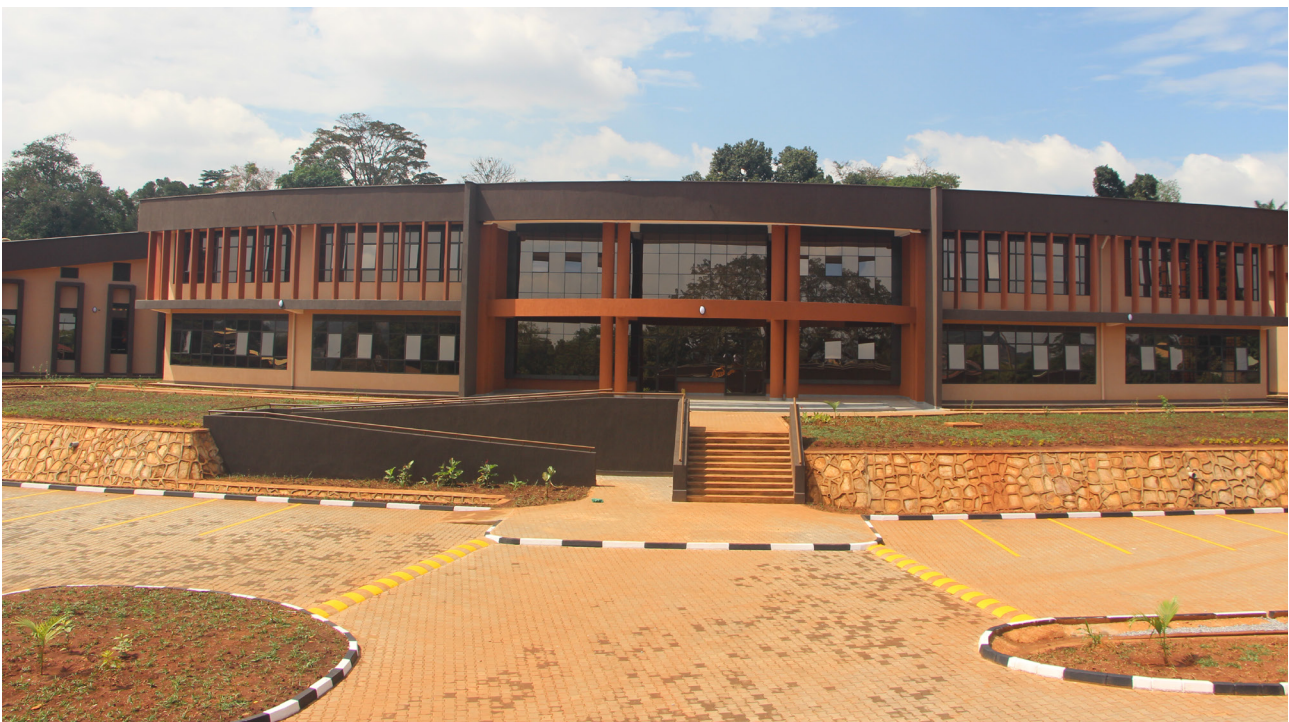
CTF Building - Kyambogo University
